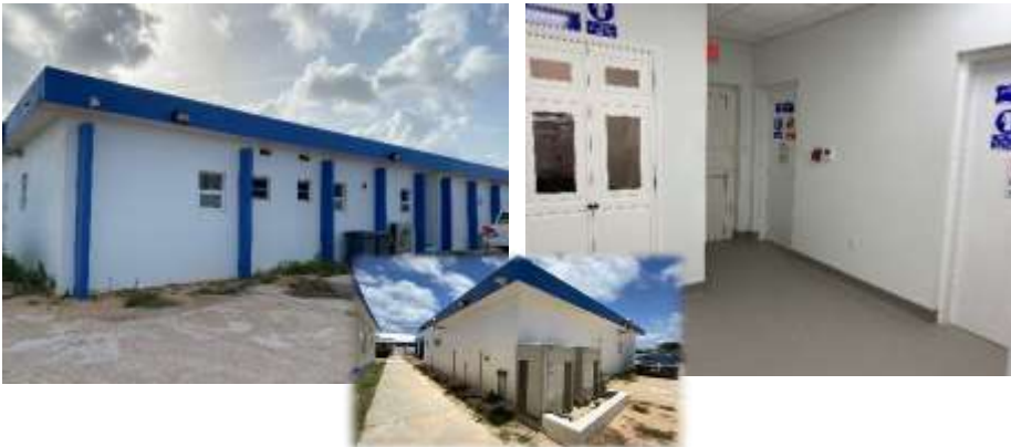
(Left) Exterior of Laboratory expansion -Eastern side view, (Centre) Western side and back view and (Right) A section of the inside of the Laboratory expansion.
